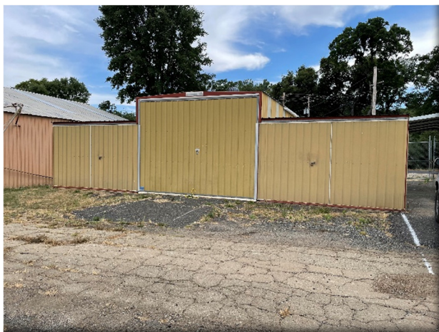
Portable T-Hangar Richard
